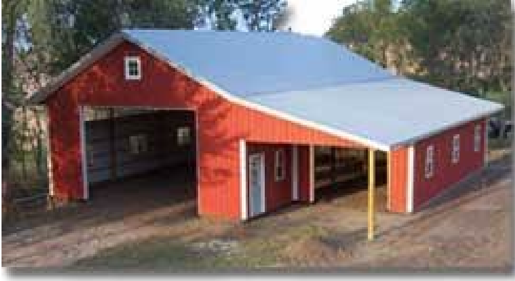
Wood frame construction type D / Average class (DA)
