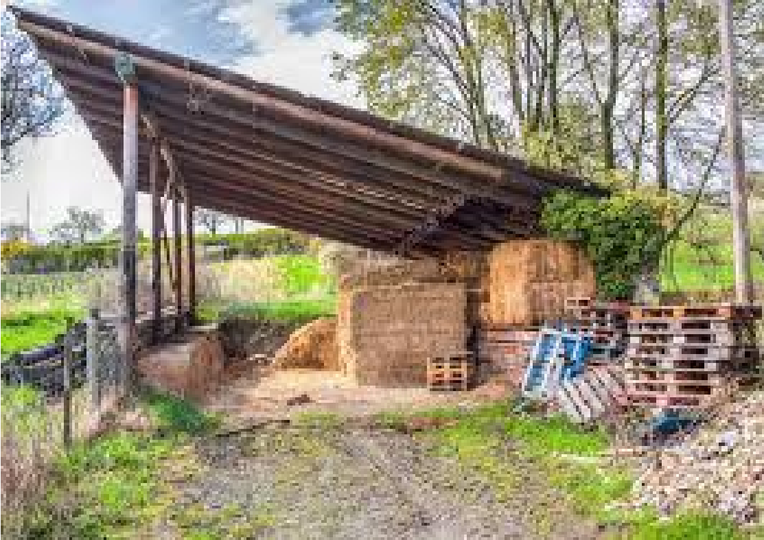
Wood frame construction type D / Average class (DA)
