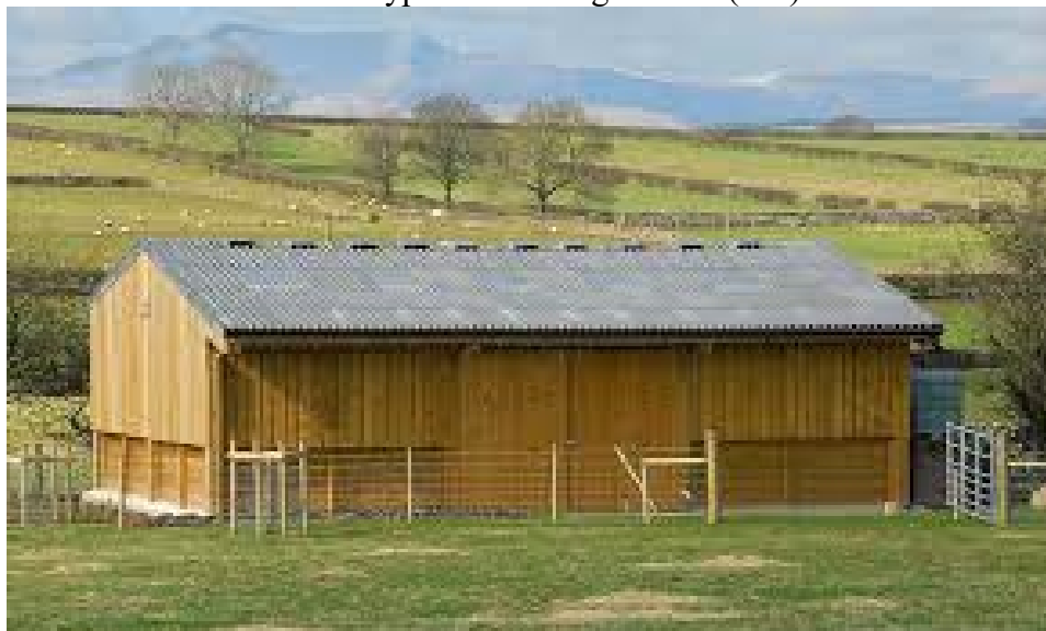
Wood frame construction type D / Average class (DA)
