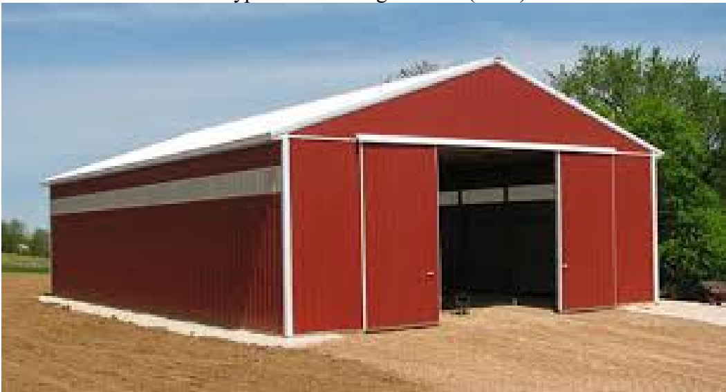
Pole construction type DP / Average class (DPA)
